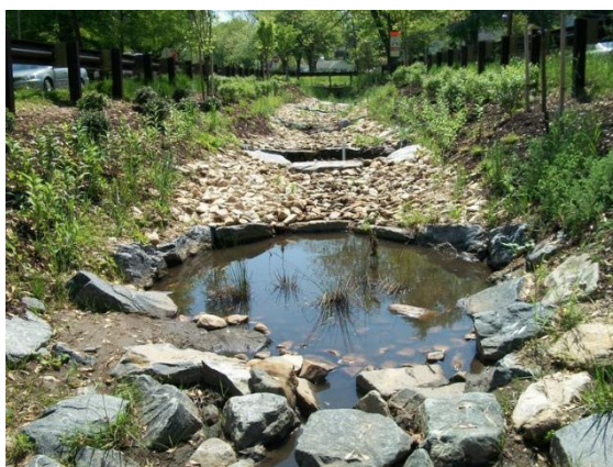
Figure 6.10 Loose Stone Check Dam
