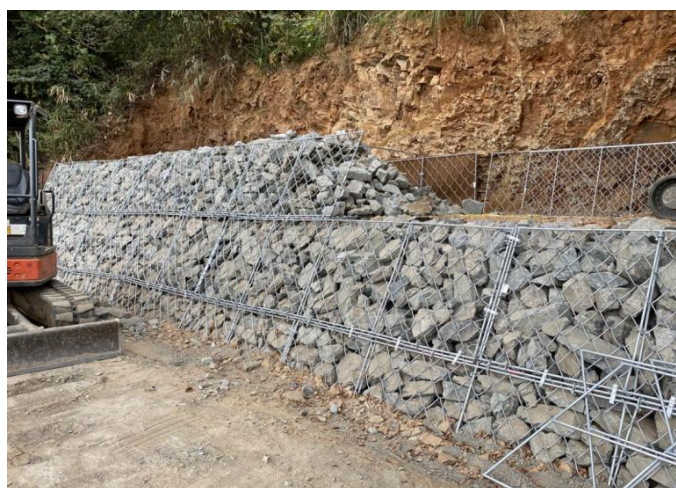
Figure 6.11 Gabion Check Dam
